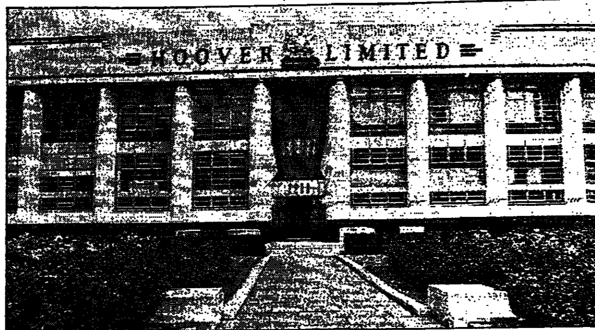
"If it's stationary, list it?" Thirties factory to early pillarbox - all come to the attention of English Heritage
